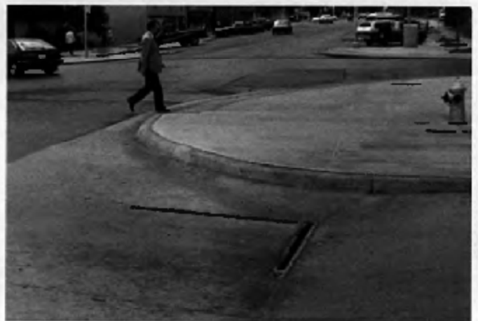
Barlesville, Oklahoma required an urban installation which could collect the flow in two directions, allowing pedestrians greater access to the crosswalks. The installation also provides an additional safety factor should a newspaper or debris cover part of the openings.
