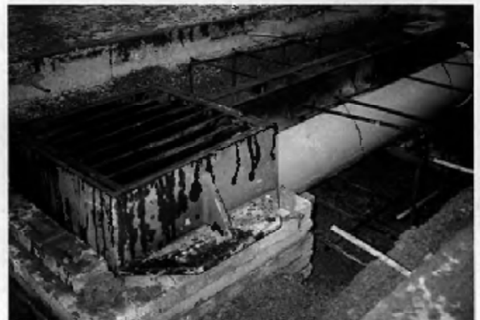
The advantages of utilizing the Slotted Vane Drain are numerous: 1) Cast gray iron as a material offers durability,
